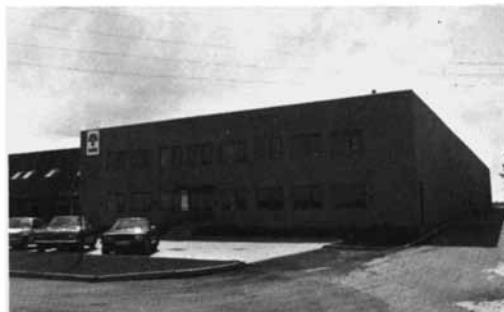
Figure 11. Development center in the dairy industry (outside)
